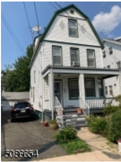
Front View Front with Driveway
