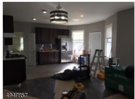
kitchen in progress
