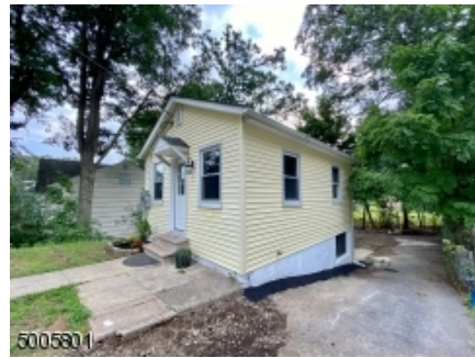
Driveway is coming
