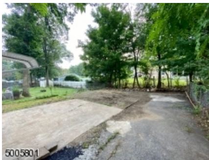
Driveway is coming
