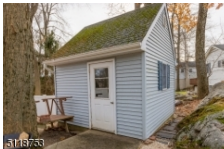
Shed / Workshop Electric
