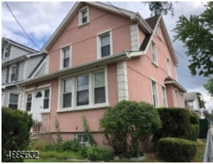
Front Right View Newer Roof, Stucco Exterior
