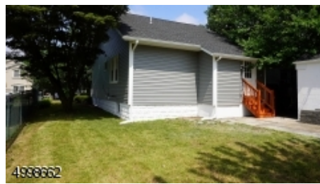
Rear of Property/Garage
