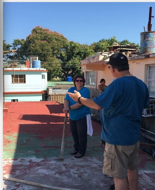
(Above) Work on the roof of the Juanelo church parsonage.
