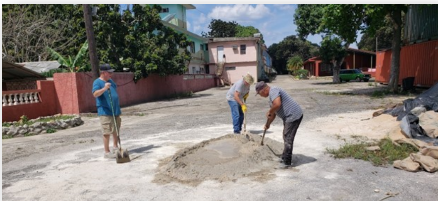
(Above) Concrete work at the seminary.
