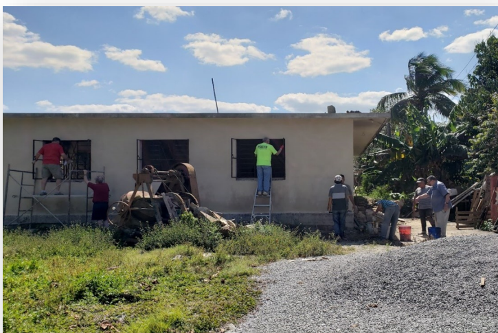
(Left) Tedious work on these windows.
