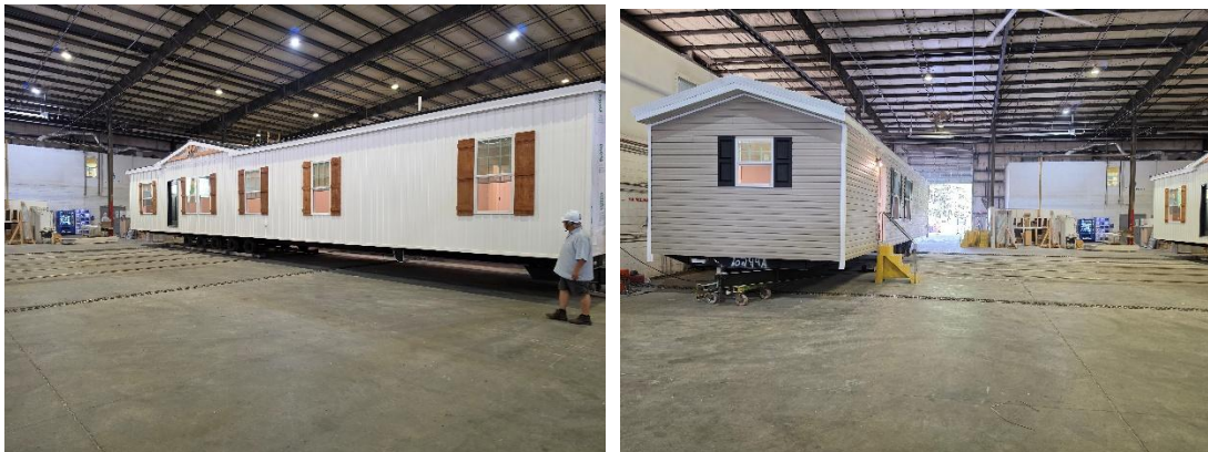
Windows, siding and other exterior finishes were added during later stages before the home left the plant.
