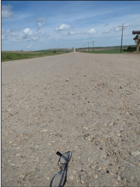
enzyme stabilized gravel – stage 1
