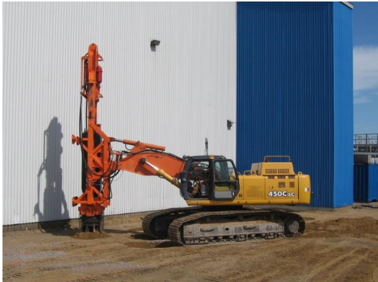
Rapid Impact Compaction
