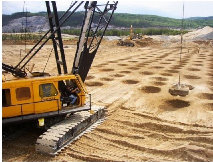
Dynamic Compaction
