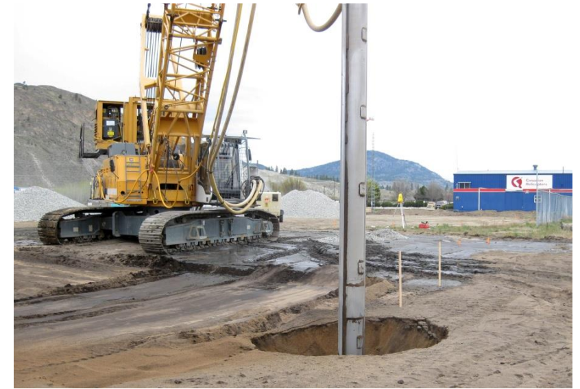
Vibro Compaction
