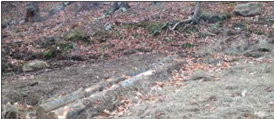
Example of log reinforced water bar on active harvest. Photo credit: Vermont AMP Manual
