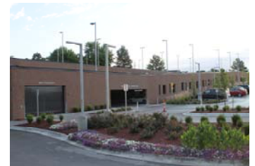
Parking Garage HCA Overland Park Regional Hospital Overland Park, KS
