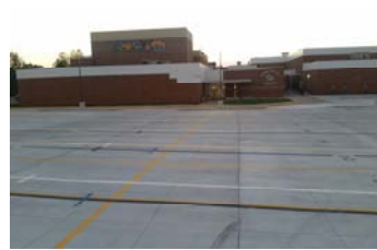
Parking Lot Blue Valley High School Stillwell, KS
