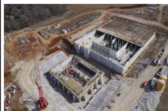
Infrastructure Hedge Lane Pump Station & Reservoir, Olathe, KS
