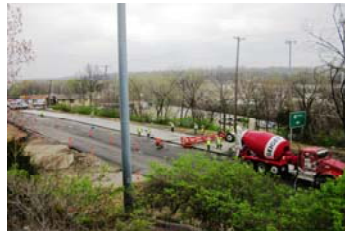
Municipal Paving Merriam Lane Kansas City, KS
