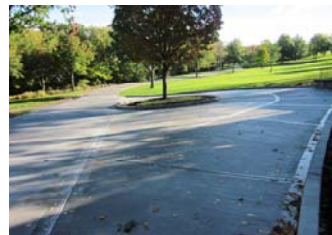
Residential Concrete Smith Residence Kansas City, MO
