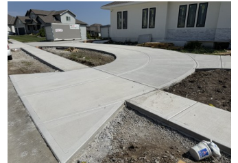
Residential Exterior Flatwork Hemayoun Residence Overland Park, KS
