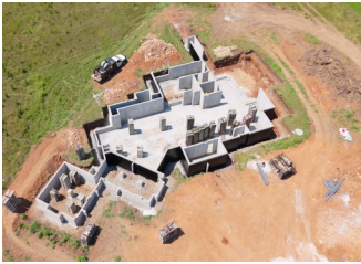
Residential Foundation Private Residence Stilwell, KS
