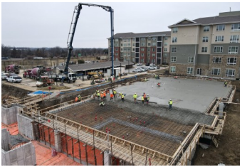
Multifamily Tallgrass Creek RB 2.3 Overland Park, KS
