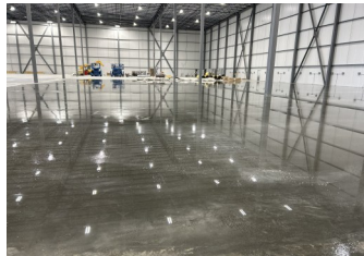
Commercial Interior Floors New Century Cold Storage New Century, KS
