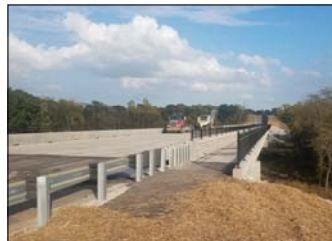
Bridge South Liberty Parkway Ph. II Liberty, MO
