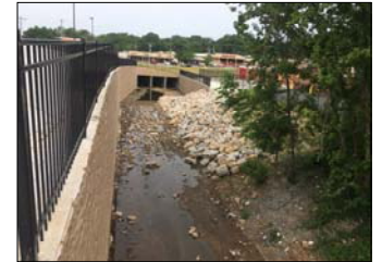
Infrastructure Nieman Storm Drain Improvement Shawnee, KS
