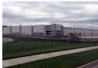
Site Cast Tilt-Up KCI Logistics Park Bldg #4 Kansas City, MO
