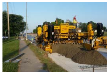
Paving/DOT Metropolitan Avenue Leavenworth, KS
