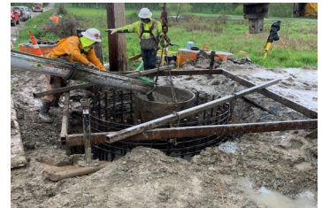
Specialty Drilled Shaft Foundations 69kV Transmission Line Rebuild Warrensburg, MO
