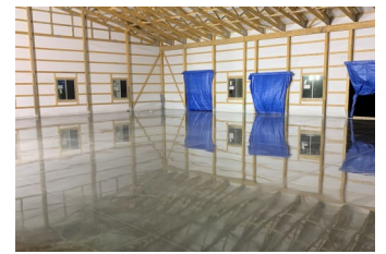
Polished Concrete DeSoto Shop Floor DeSoto, KS
