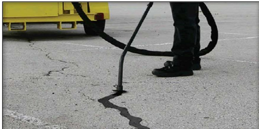
**Purpose:** The purpose of sealing and filling cracks in the pavement surface is to prevent water and incompressibles from entering the pavement structure.
