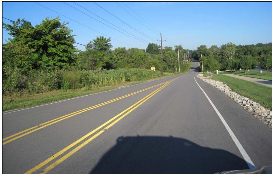
**Purpose:** A single course micro-surfacing will retard oxidation and improve skid resistance in the pavement surface. A multiple course micro-surfacing is used to correct certain pavement surface deficiencies including severe rutting, minor surface profile irregularities, polished aggregate or low skid resistance and light to moderate raveling. Micro-surfacing is typically used on flexible or composite pavements and can perform under all traffic volumes.
