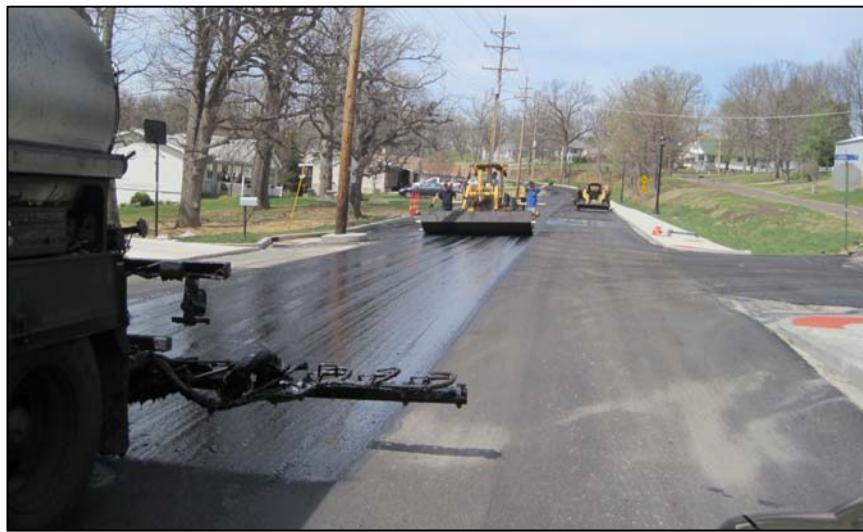
**Asphaltic Surface Course** - The bituminous overlay replaces the bituminous material that is removed.
