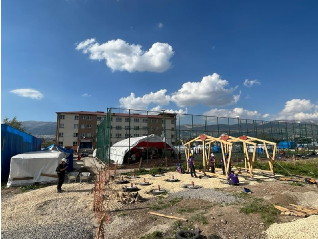
Volunteers work on constructing a women's and infants' commons area, with an existing school in the background (which was evaluated for safety). Photo courtesy Paul Brallier.
