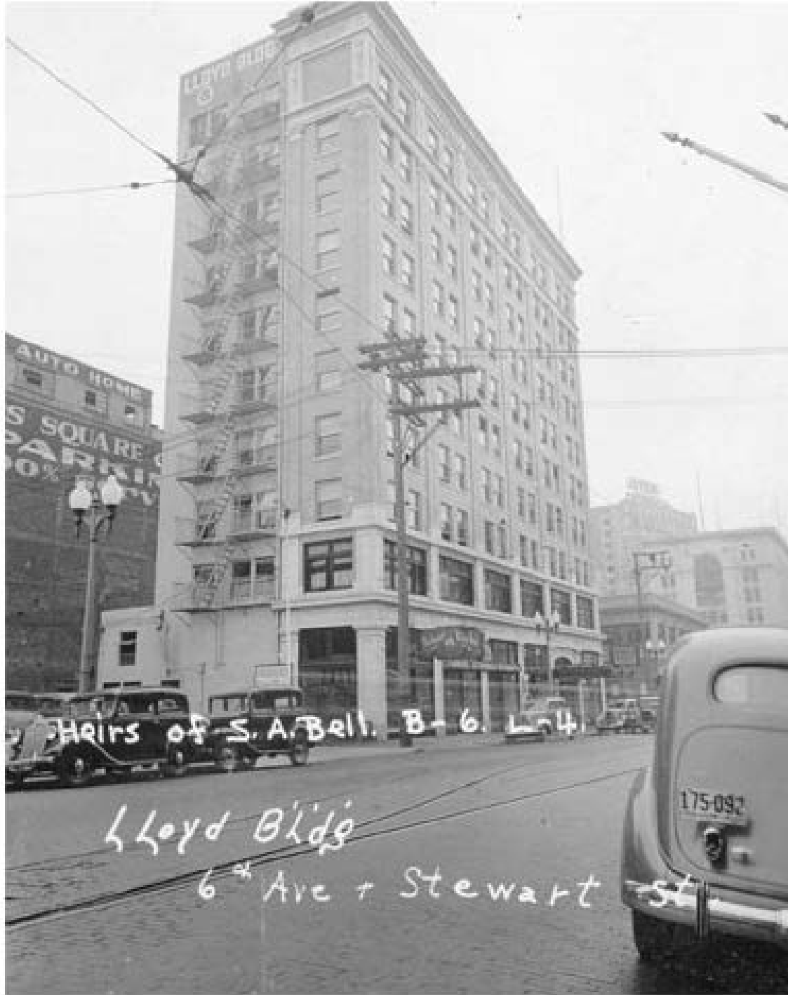
The Lloyd Building, a 10-story building in Seattle, was completed in 1928 and held offices of one of the city's first structural engineering firms. Image courtesy the MKA website.
