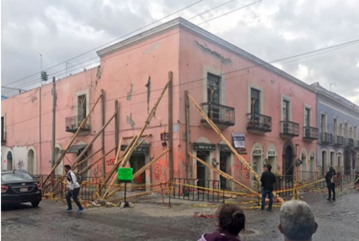
Shoring of an unsafe building in Puebla, Mexico, damaged by the 2017 Central Mexico Earthquake. Photo courtesy Erik Bishop.
