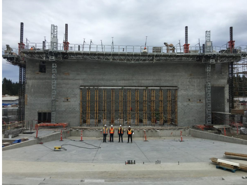
Reinforced concrete masonry beam with a clear span of 48 feet and 20 feet tall. Ian Kane, Morgan Wiese, Casey Moore (who designed the beam) and Ben McElroy. Credit: Tom Corcoran
