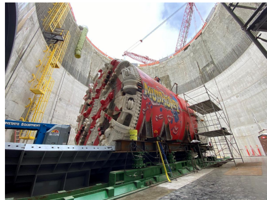
“Mud Honey” is a tunnel boring machine which made a nearly 19-foot hole for 2.7 miles underneath multiple Seattle neighborhoods. Photo courtesy Keith Ward.
