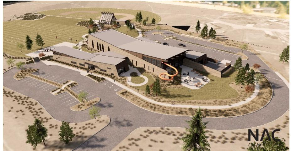
Construction consists of a combination of heavy timber framing with SIPS roof panels, conventional wood framing, and concrete masonry units.
