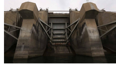
The Wanapum Gates is an example of tainter gates on dams, which the South Central Chapter learned more about in February. Photo provided by Matt Leslie.
