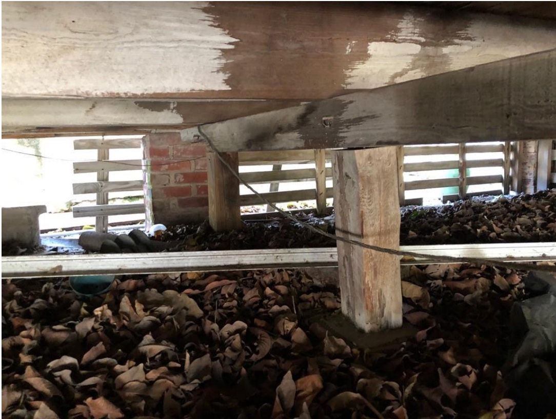
BEFORE: Vestry Room held up by 4x4 and tree trunk.
