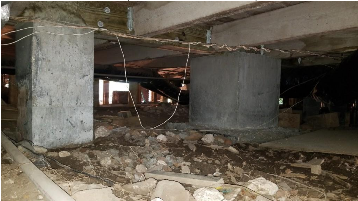
AFTER: New Reinforced concrete pillars with new beams attached by steel brackets
