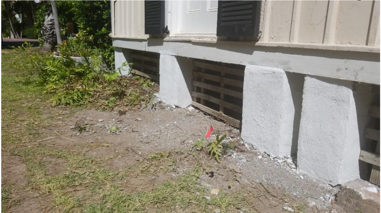
AFTER: Visible Pillars repaired as needed and made uniform with protective stucco coating
