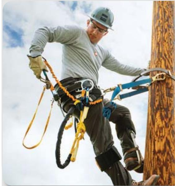
Another often overlooked fall protection topic is dropped object prevention. A utility pole worker climbing a pole uses a tool lanyard for dropped object control.
