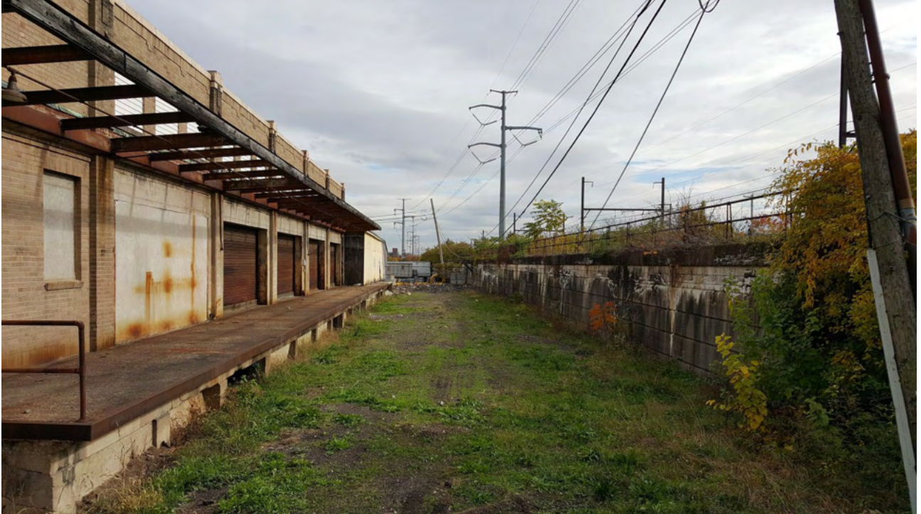
South side of building before construction, looking east.
