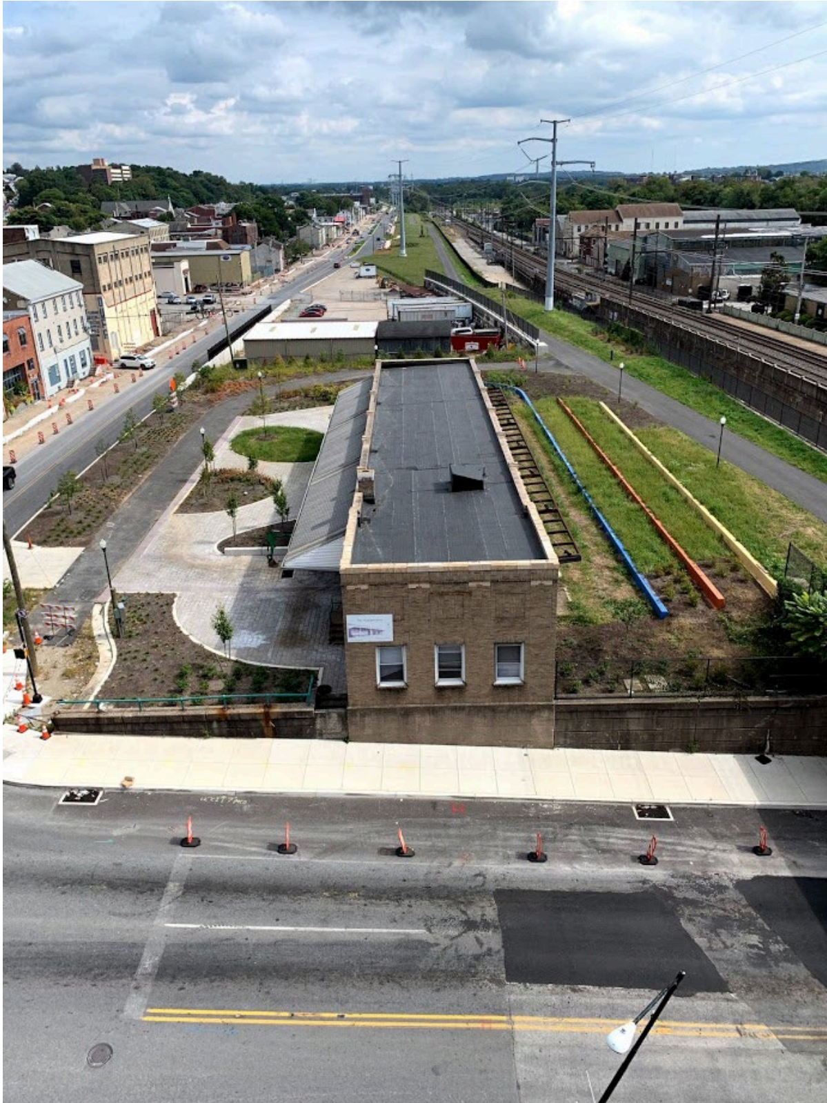
Trail Junction Center and site following site improvements in 2019.
