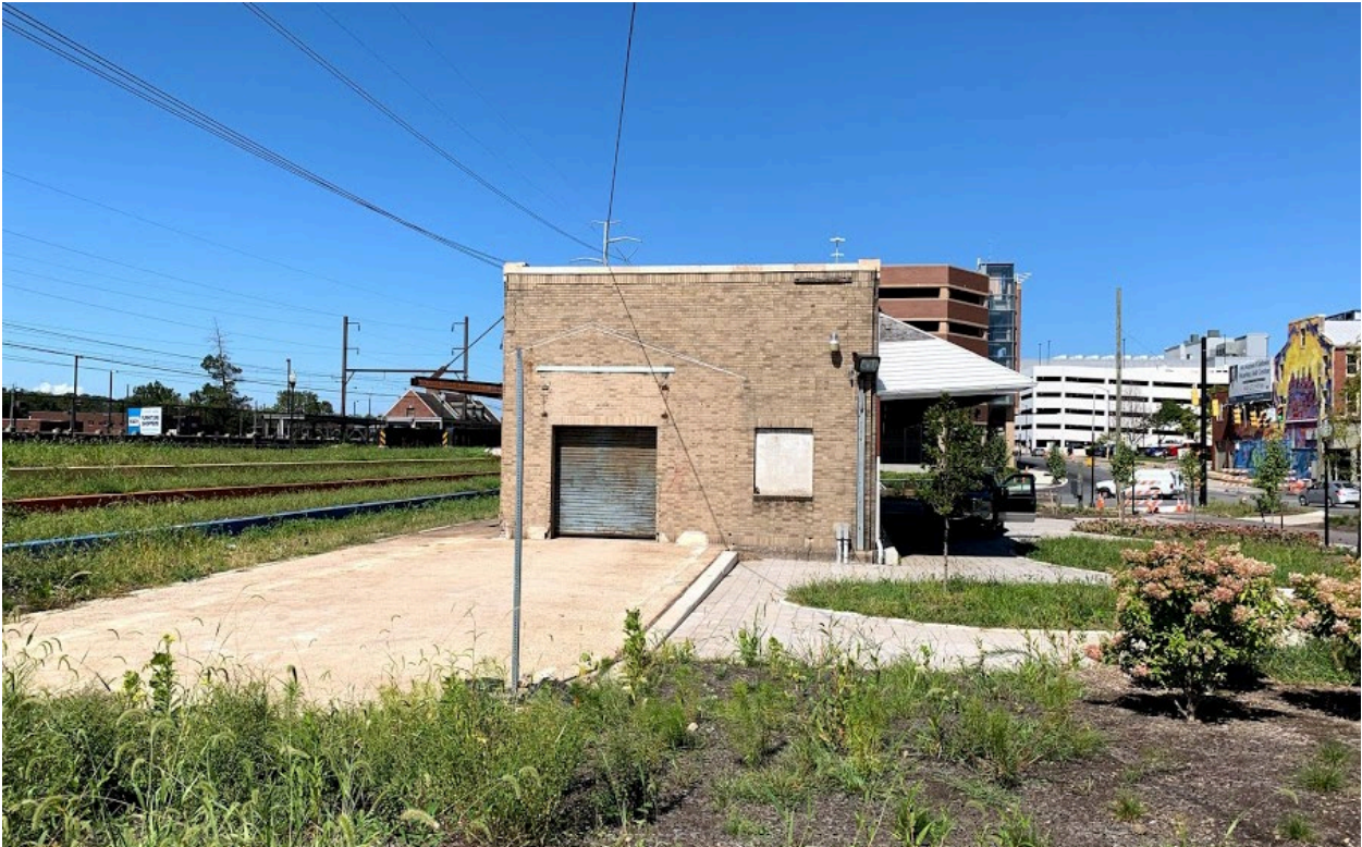
East end of building following site work.
