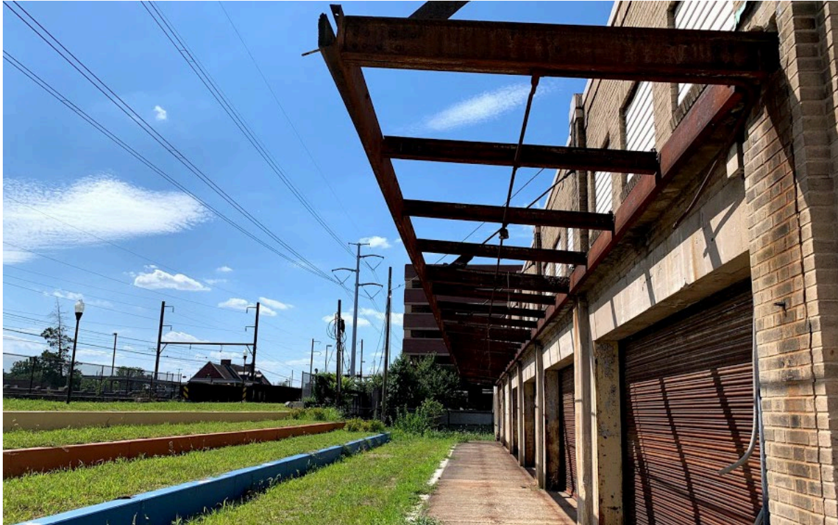
South side of building.
