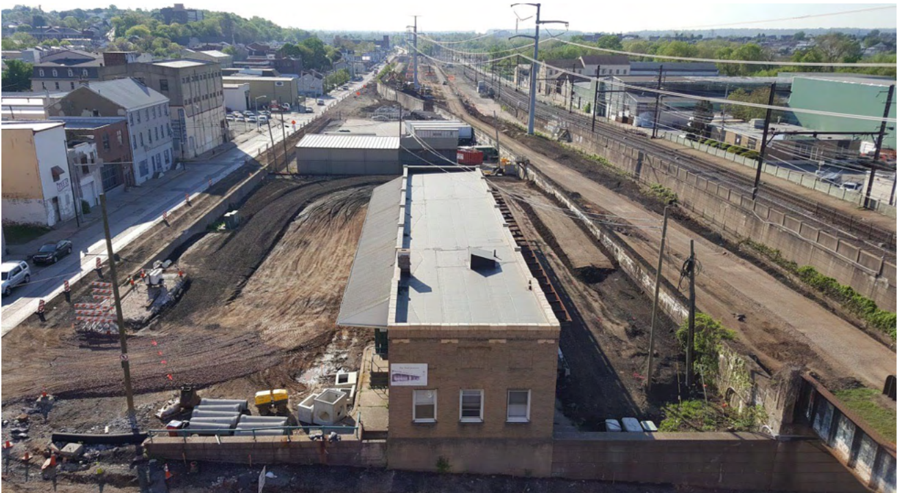
Aerial view of building during site work construction.
