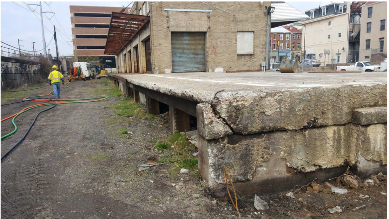
South side of building during construction, looking west.
