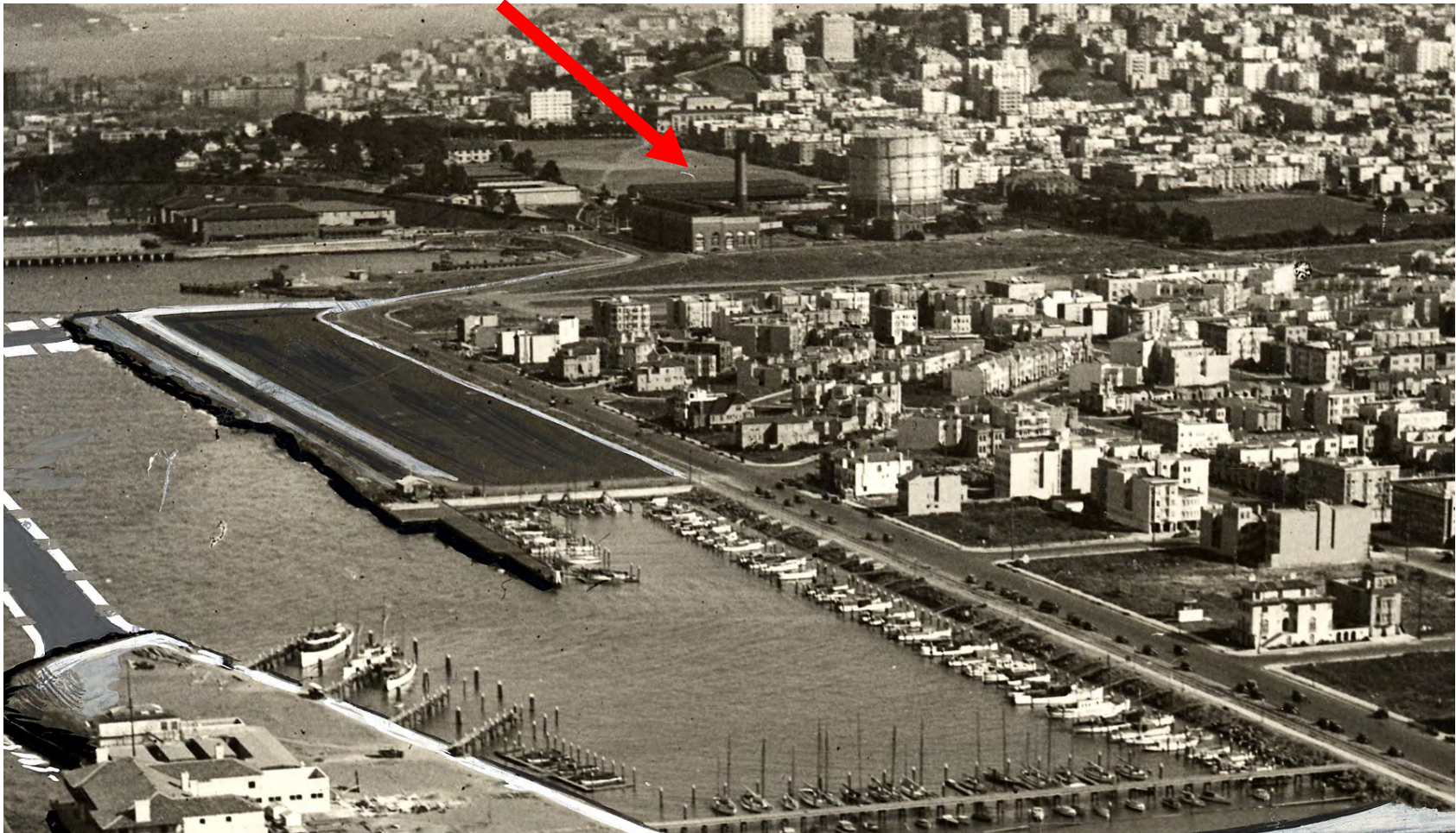
Figure 11: May 27, 1929, Detail view looking southeast. Source: SFPL History Center AAB-9432.
