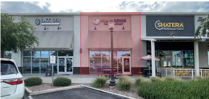
BUILDING B2 - 1,141 SF In-Line Space Available (tenant in place, available upon negotiation)
