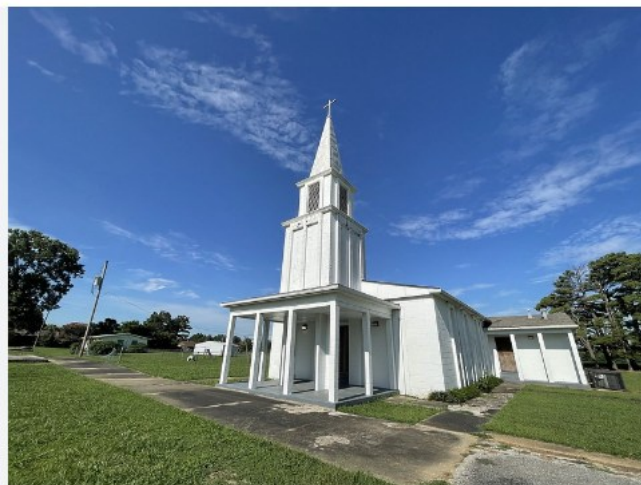
Christ Episcopal Church's chapel and parish remain a landmark in Forrest City, Ark.
