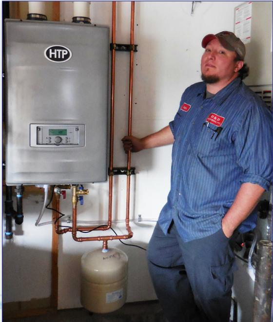
Tina McKendree, the bookkeeper at D&D Plumbing, Inc. in Sparks NV, recently had an HTP RGH-199 Crossover water heater installed, replacing the original 50 gallon natural gas water heater. A Taco HotLink thermal by-pass valve was installed at a bathroom sink. There are currently 3 adults and 3 teenagers living in the house.
