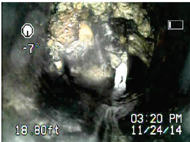
Photo 5 - The drain line is over 80% clogged.
