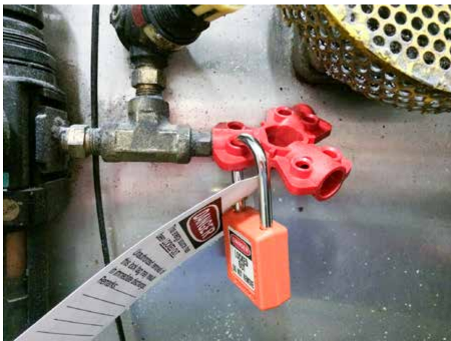
Lock on a pneumatic disconnect as part of a compressed air energy source
