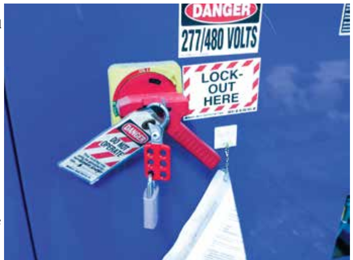
Lockout/Tagout for electrical power source for grinding machinery
