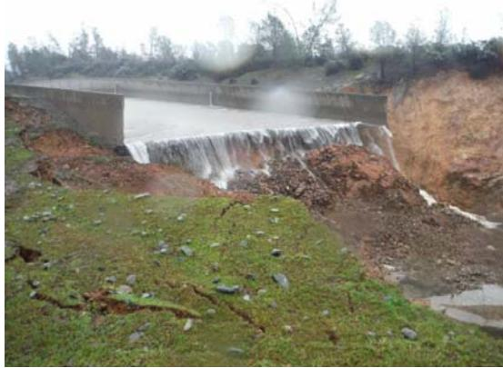
EagleLIFT's Scan and Repair approach is a cost-effective method for identifying issues and then repairing the problems quickly and cost-effectively. Firstly, detecting the problem is the main focus. For this we utilize a Ground Penetrating Radar (GPR) system to scan the entire spillway and determine if there are any voids present. If voids are present, we then fill the voids and stabilize the
