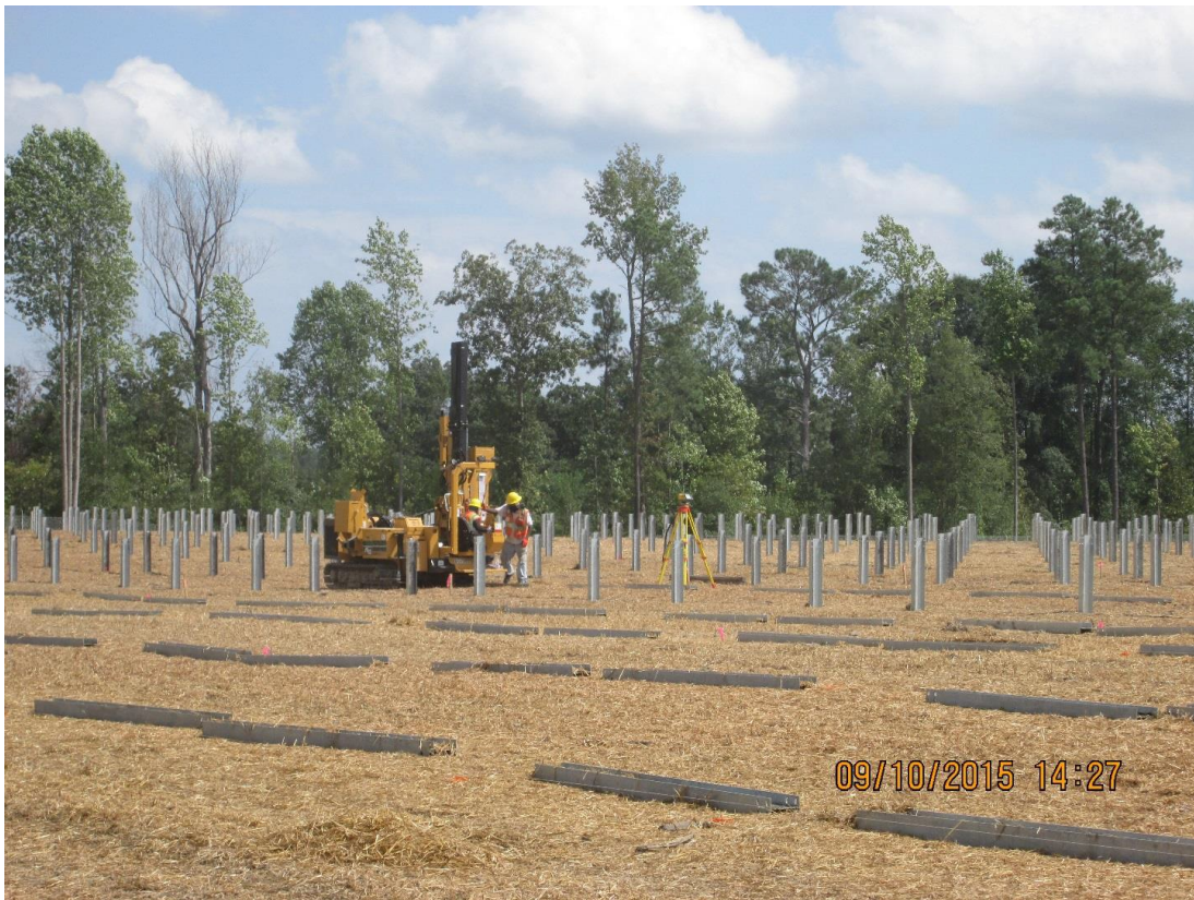
Good staged seeding and mulching between grading and pole installation. Photo courtesy of NCDEQ
