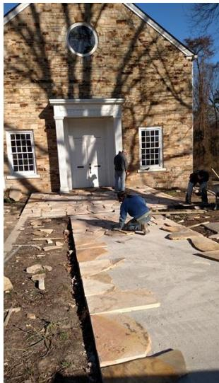
The front walk and patio, as well as the sidewalks leading to the side-door entrances, are being completely renovated. Years of deterioration and damage from tree roots rendered the stone walkways hazardous. New stone walks will be sloped for better drainage and accessibility purposes.
