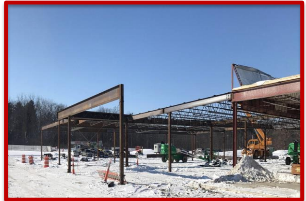
Picture 1: Structural Steel Erection – East View looking West
