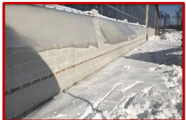
Picture 3: Masonry Veneer at Southern Elevation
