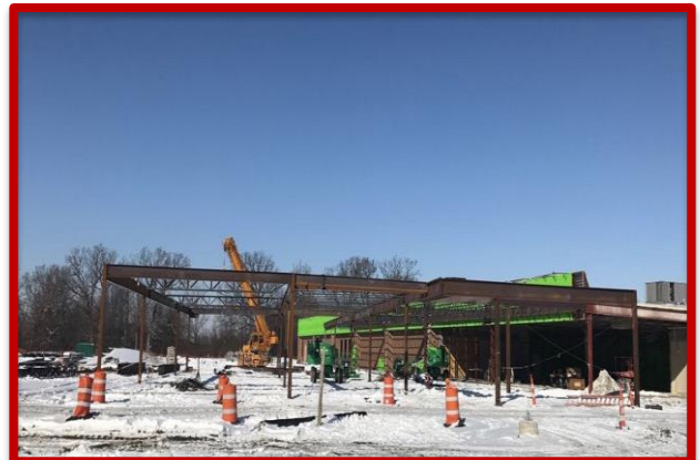
Picture 2: Structural Steel Erection – South View looking North
