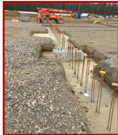
Picture 2: Progress on the firewall foundation between Automotive and Student Dining
