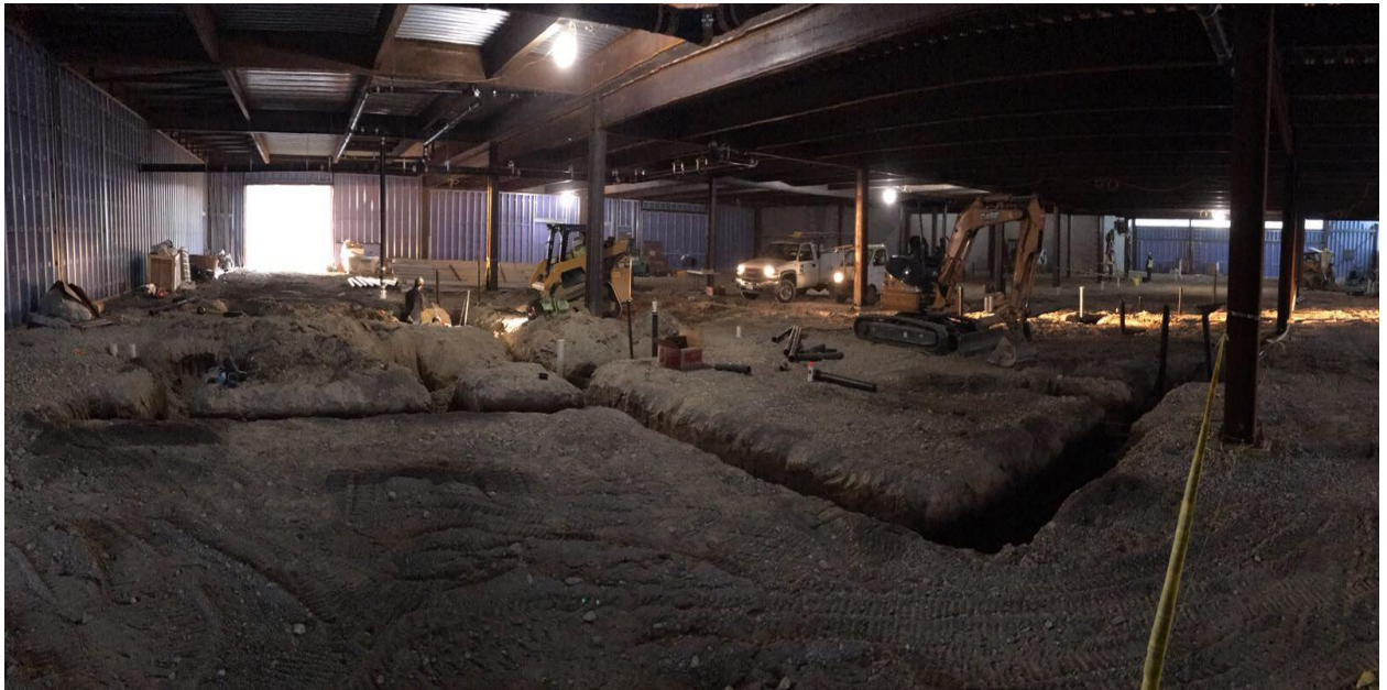
Picture 6: Underground Piping Installation in Area D and E.
