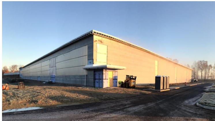
Picture 2: Southwestern Elevation Exterior Insulation
