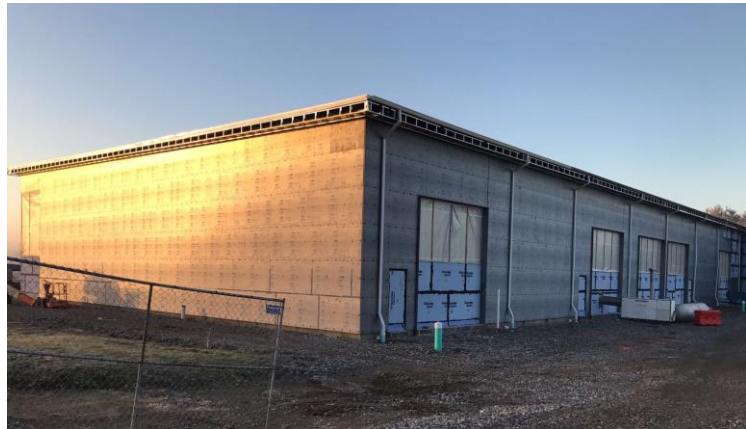
Picture 1: Southeastern Elevation Exterior Insulation
