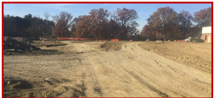
Picture 3: Grading of site along north west end of site
