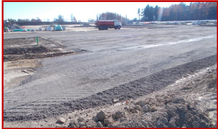
Picture 1: Placement of stone for building pad
