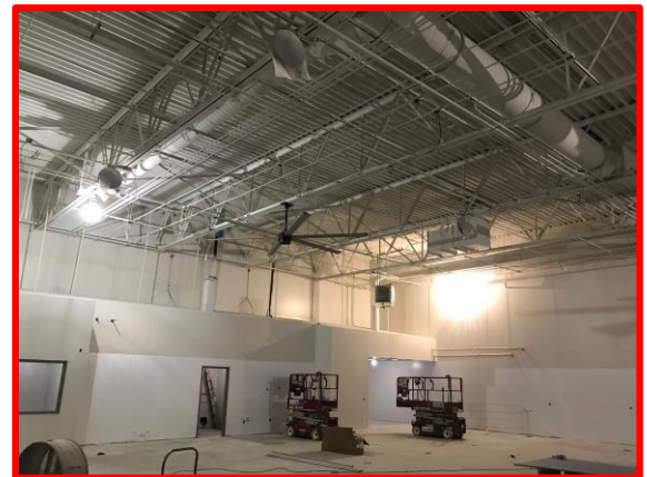
Picture 3: Progress in Construction Tech Lab
