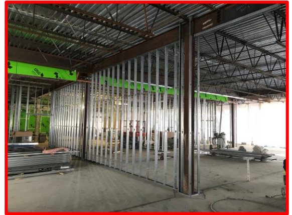
Picture 1: Metal Framing Progress in Admin Area
