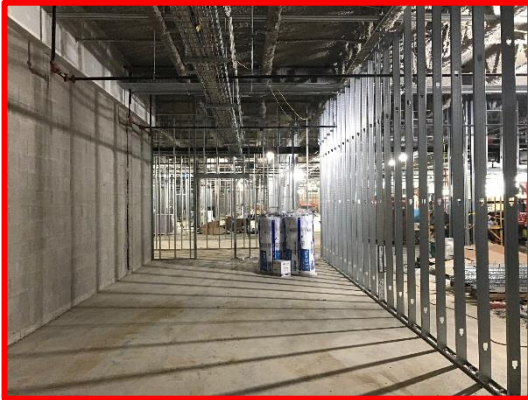
Picture 1: Interior Framing in the Teacher Prep Room in Area H
