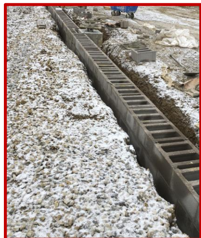
Picture 3: CMU foundation progress in Area A
