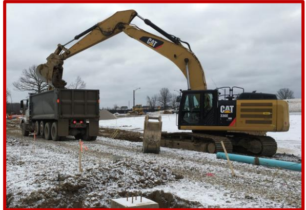
Picture 1: Waterline installation ongoing
