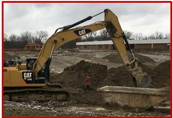
Picture 2: Fire hydrant installation and backfill
