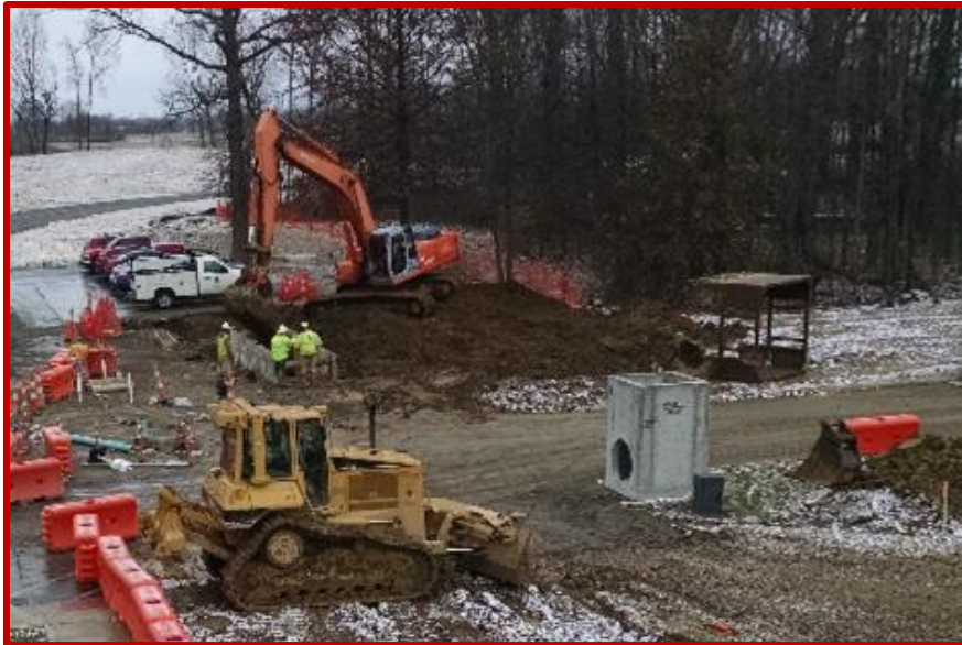
Picture 4: Installation of storm structures on the north side of campus
