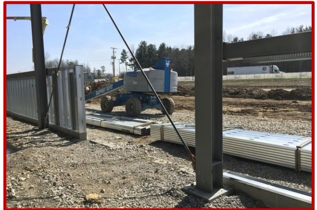
Picture 2: Metal stud framing through cross-bracing in Area C
