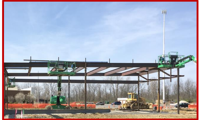
Picture 1: Structural steel progress in Area E's LG Conference Room
