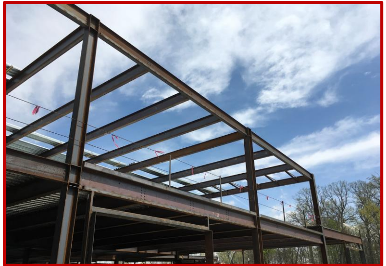
Picture 5: Progress on Area E's second floor structural steel awaiting decking
