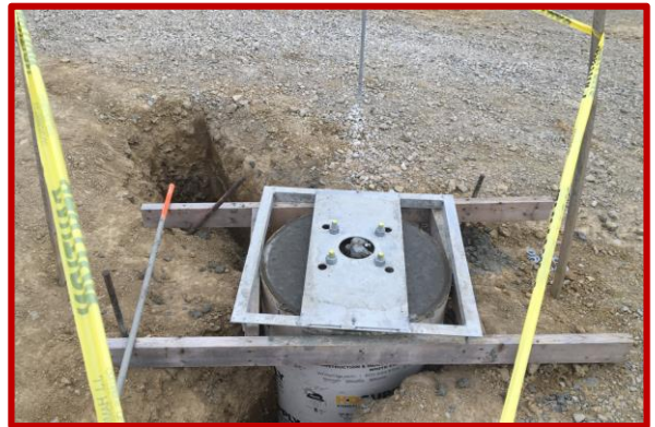
Picture 2: Concrete formwork for a light pole base in the South Parking Lot
