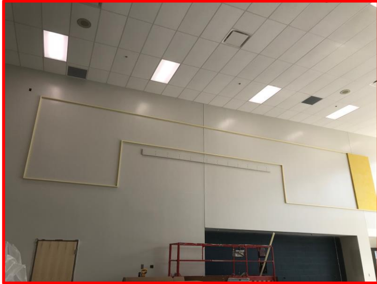
Picture 4: Prep for Acoustical Panel Installation in Student Dining
