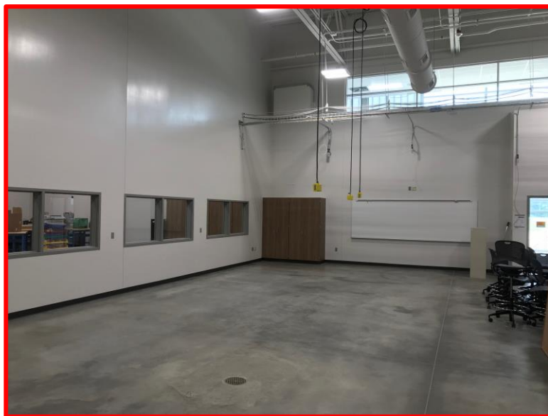
Picture 5: Electrical Drops in Engineering Tech High Bay Lab
