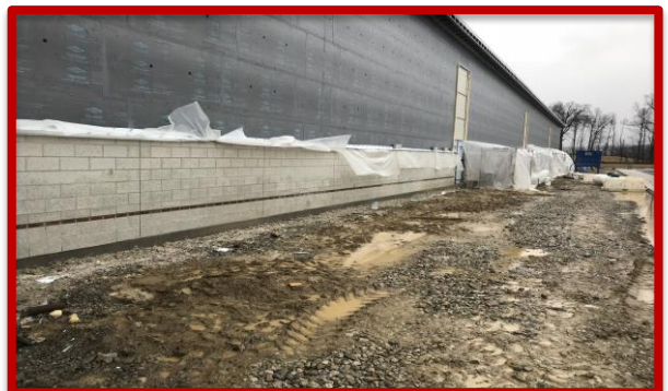
Picture 3: Masonry Veneer at Southern Elevation
