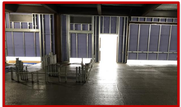
Picture 2: Slab on Grade section poured in Area E
