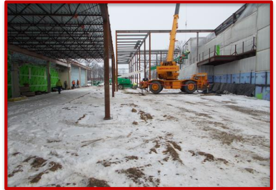
Picture 1: Steel Erection at Building Connector
