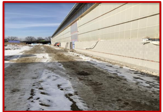
Picture 2: Installation of Masonry Veneer at the West Elevation
