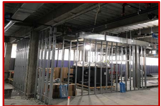
Picture 3: Interior Framing in Electrical Room near Student Dining Area
