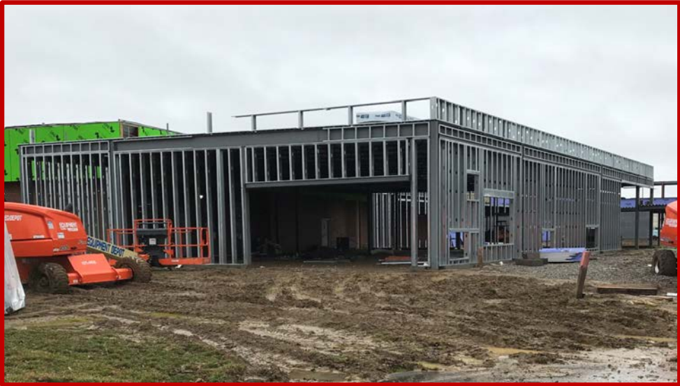
Picture 5: Exterior Framing of Early Childhood Development Area
