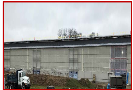
Picture 2: Window Framing at West Elevation
