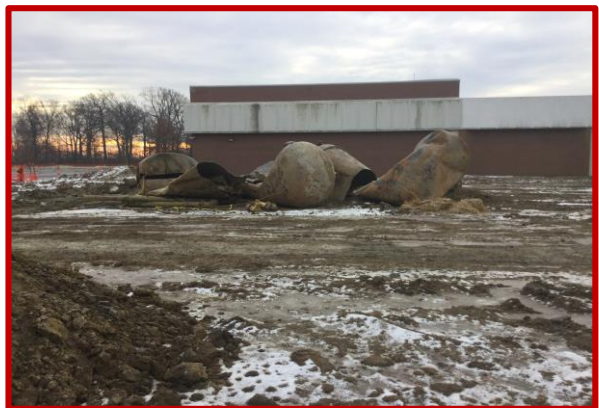
Picture 3: Storage tanks to be disposed
