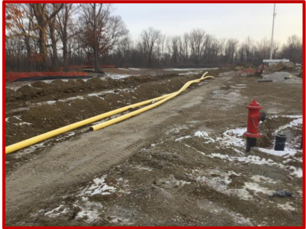
Picture 1: Progress on gas line installation
