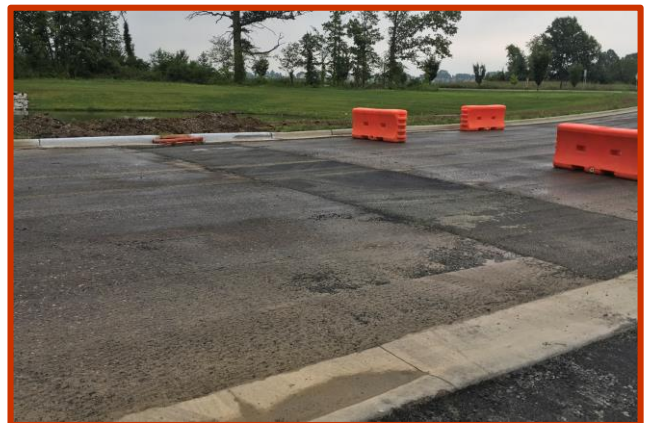
Picture 3: New curbs and gutters on the newly milled Peachblow Road
