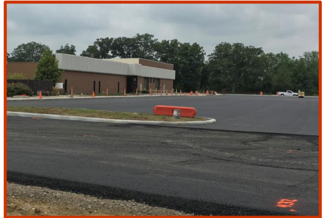
Picture 1: Asphalt pavement progress in the existing East parking lot
